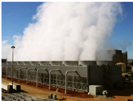
Fig. 2. Plumes rising from an 18-cell mechanical draft cooling tower. The cells are arranged in two rows of nine cells [photo from Marley, 17].
