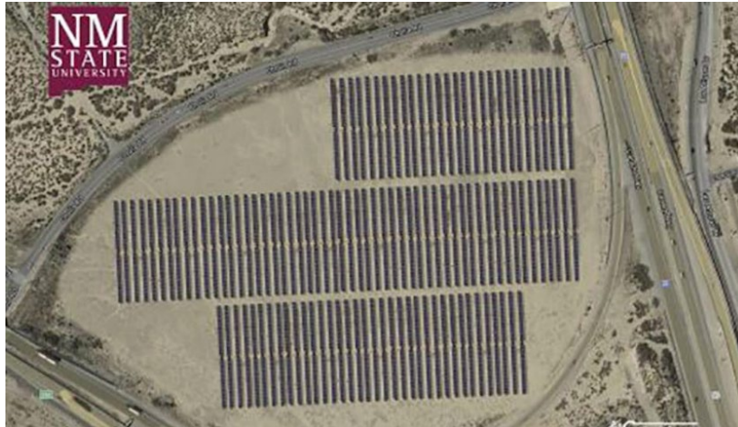
Fig. 1. Aggie Power facility, aerial view. Desert plants line the outside perimeter of the facility.
